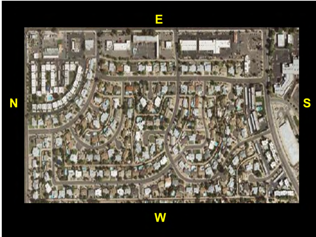
This contemporary aerial photograph shows the totality of the Cavalier Hills and the commercial lots incorporated into the development. Cavalier Hills homes feature large lot sizes, mature vegetation, and largely intact historical integrity.
